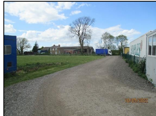
Access Track off Highgate
